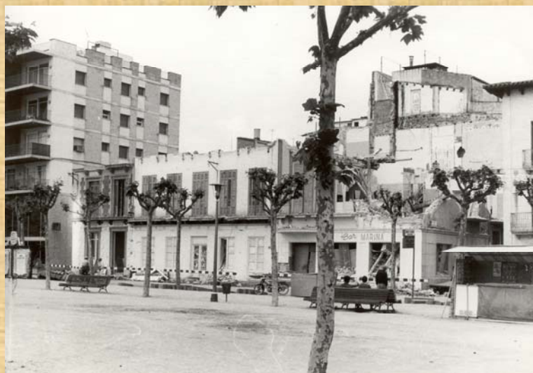
Enderroc del Restaurant Bar Marina, 1972 (AMSFG, Fons Jordi Rabell. Autor: Jordi Rabell)
